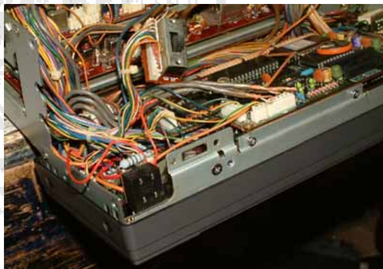
After switch removed (note that the wires are long enough that the switch can be tied back out of the way.)
