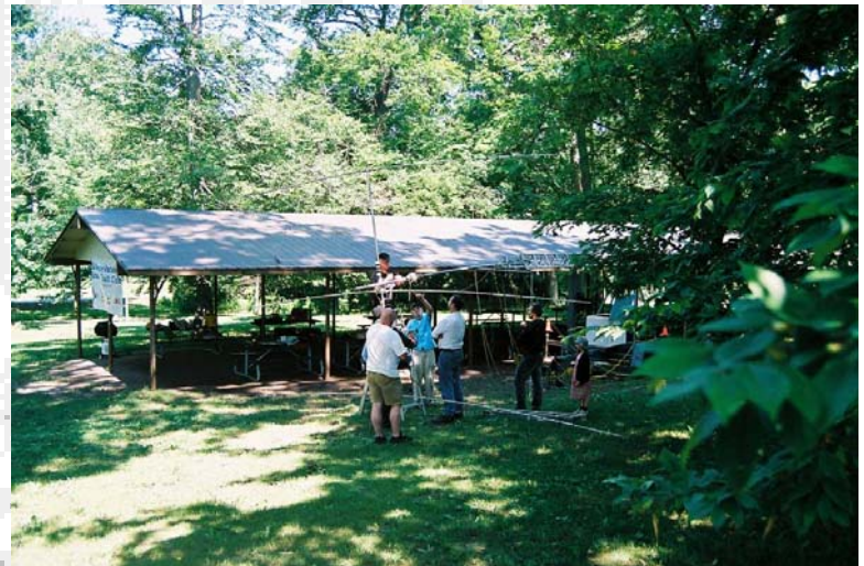
Putting The Beam On The Tower
